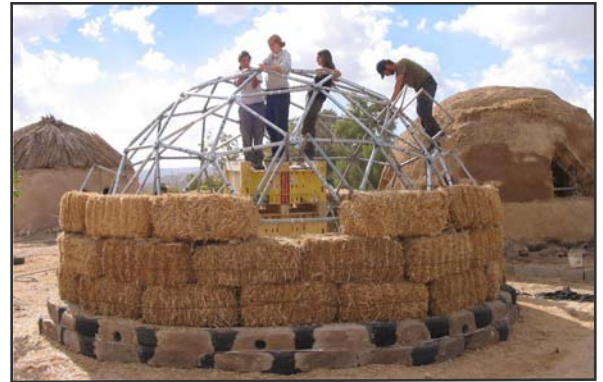
Students constructing a straw bale and earth geodesic dome
