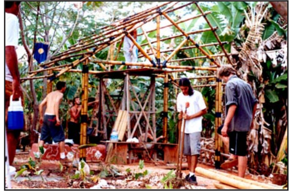
Students study and practice natural building and ecological design techniques.
